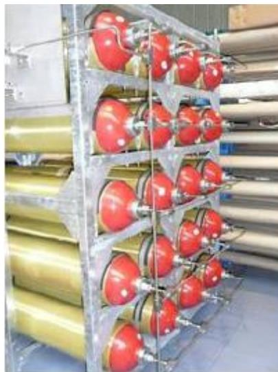
Figure 2. Buffers for hydrogen refuelling stations.
