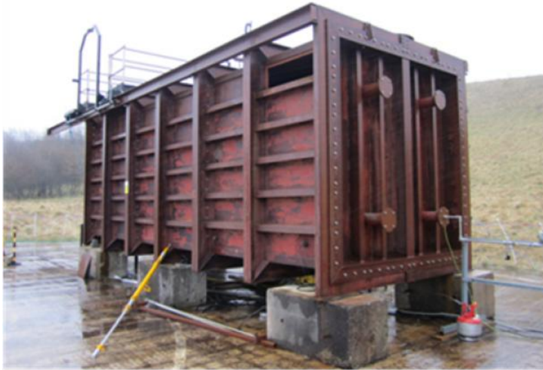
Figure 1. Exterior of the HSL enclosure with a passive vent (vent 1) open.
