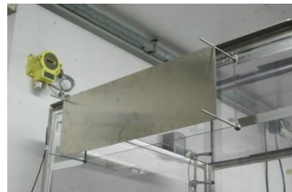
Figure 14. Vertical solid plate wind deflector placed in front of the top ventilation opening.
