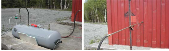
Figure 4. Gas storage tank and fuel supply system
