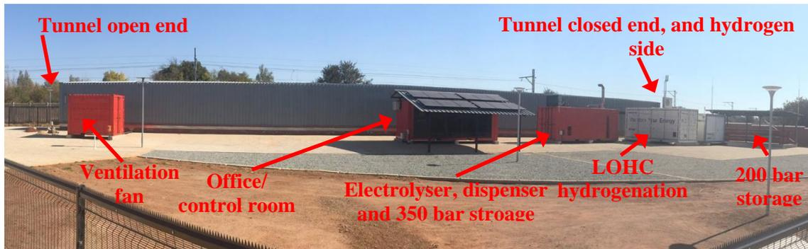
Figure 9. Ventilation test facility.
