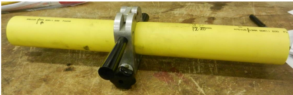
Figure 4 : Re-rounding PE80 Pipe After Completion of Squeeze-off
