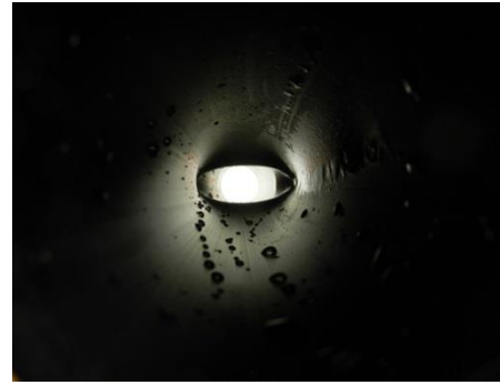
Internal view (inner walls) of pipe midway during squeeze off
