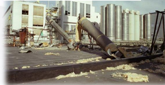
Explosion in hydrogen pipelines Norway, 1997
