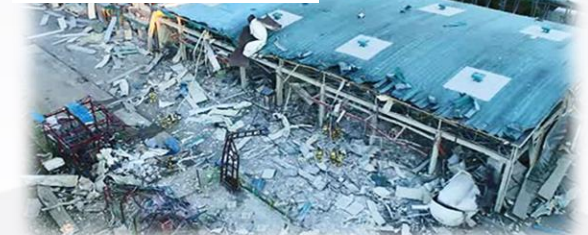
Explosion in hydrogen tank Korea, 2019
