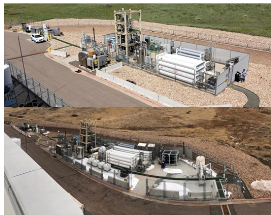
NREL HITRF Station Expansion Under IHS Project
