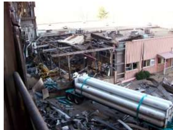
Power Plant Hydrogen Explosion Muskingum, Ohio, 2007
