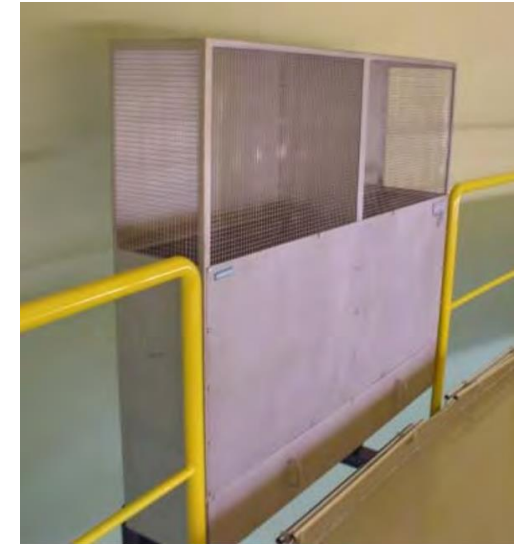
Energys-Hawker Hydrogen Eliminator
