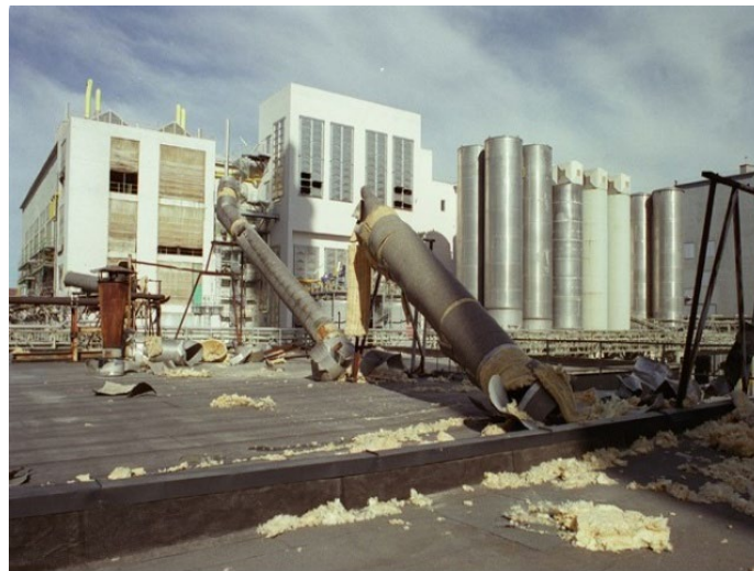
Figure A2. Flame acceleration in a hydrogen-air explosion inside a pipeline resulted in several ruptures [28]
