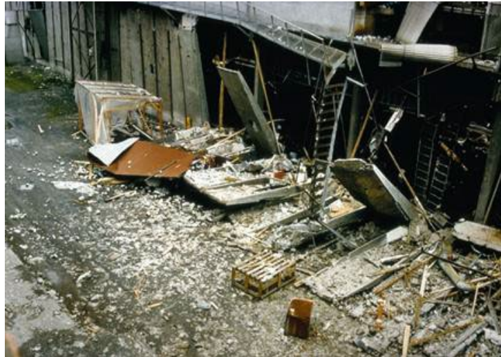
Figure A1. Damage caused by the explosion (accident investigation [27], Photo: A. Kjellevold)
