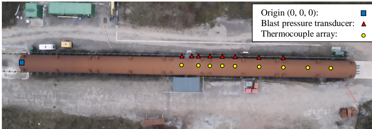
Figure 1: Overhead image showing the tunnel with sensor locations
