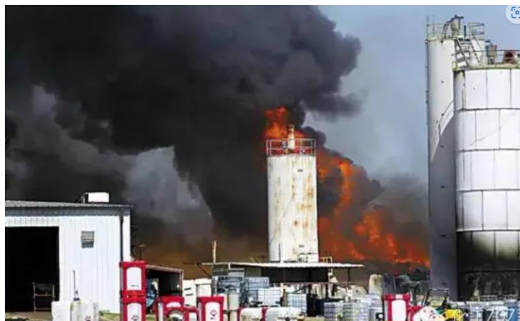
Figure 6: Accident scene after the fire (picture source: website https://www.ichemsafe.com/info/3275.html (last retrieved 20.02.2023))
