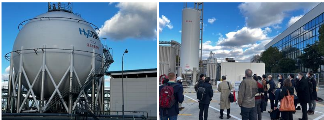
Figure 6. Liquefied hydrogen receiving terminal (left), Hydrogen co-generation system (right)
