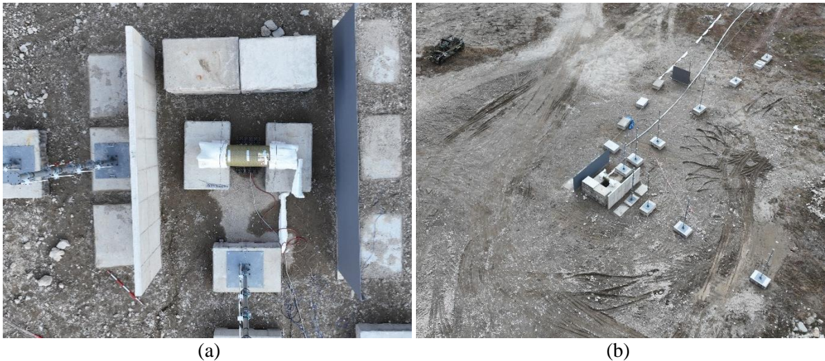
Figure 1. Experimental setting for the blast mitigation barrier against the explosion of CHSS
