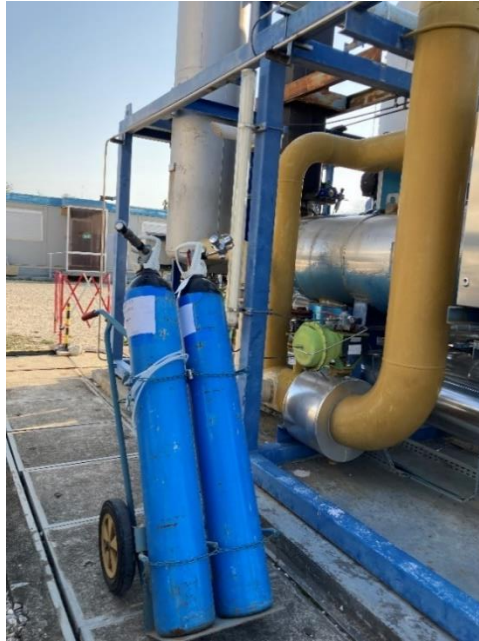
Figure 5. Air cylinders used during the tests for leak simulation
