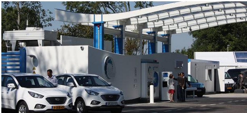
Figure 1. Hydrogen refueling station.
