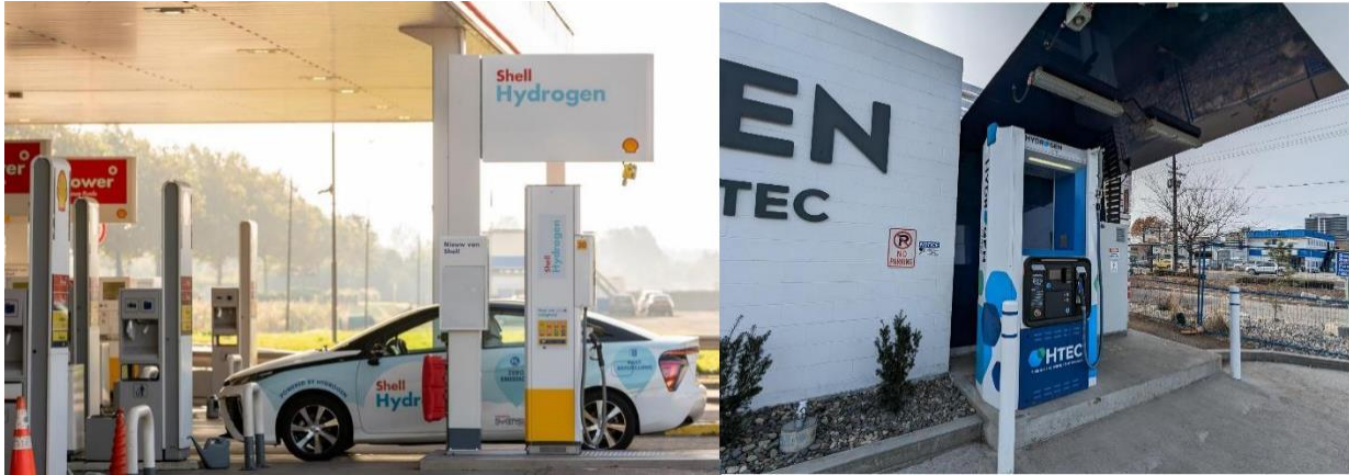
Figure 6. Left , A hydrogen fueling station integrated to a gasoline station. Right , A stand-alone hydrogen station
