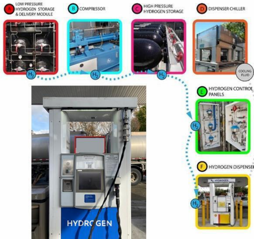
Figure 5. The major components of a hydrogen fueling station
