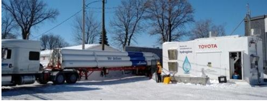
Figure 3. Hydrogen tube trailer filling a hydrogen station
