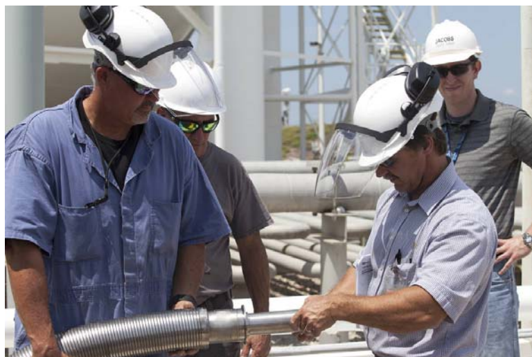
Figure 2-8. Inspection of an LH 2 supply hose at NASA's Kennedy Space Center (Photo credit: NASA/Frankie Martin).
